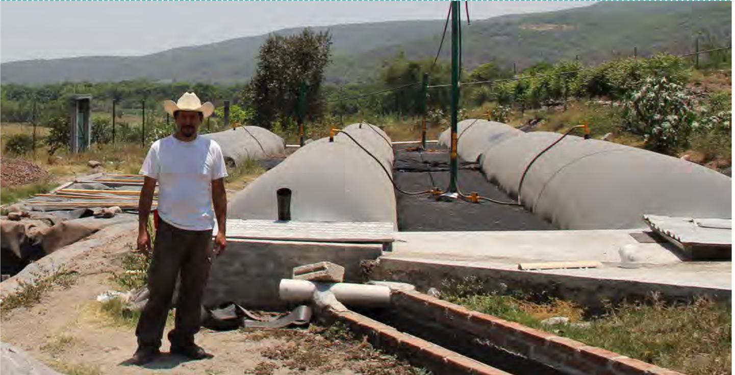
**SistemaBiobolsa®** is a patented and high quality anaerobic digestion technology that was designed to meet the specific needs of small and medium size dairy and hog farms, as well as farms with other species, for which installing industrial biodigesters is not an option. Using the waste from a wide range of animals at the farm, Sistema Biobolsa® produces clean and renewable energy that can be adapted and used to produce thermal, mechanical or electric energy.
