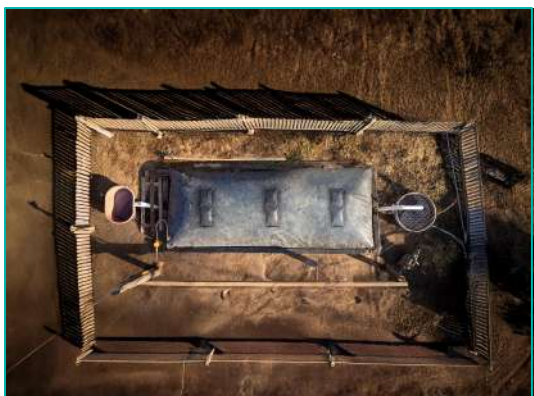
Sistema 16 Area Required: 11.5 x 4.0 m Biogas: 4.8 m 3 /day*
