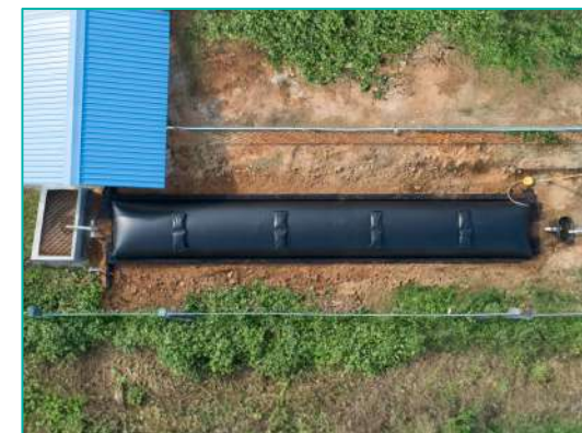
Sistema 40 Area Required: 23.0 x 7.0 m Biogas: 13 m 3 /day*
