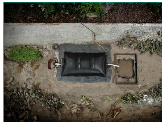
Sistema 12 Area Required: 9.5 x 4.0 m Biogas: 3.3 m 3 /day*
