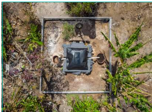
Sistema 6 Area Required: 7.8 x 4.0 m Biogas: 1.7 m 3 /day*
