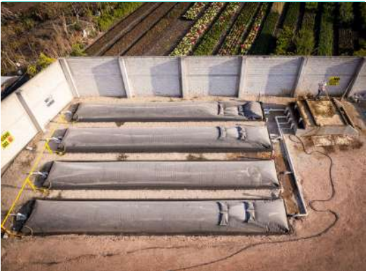
Sistema 160 Area Required: Sis 40 x 4 Biogas: 52 m3/day*
