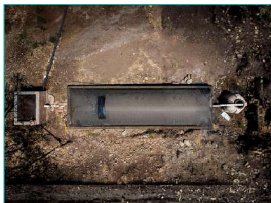
Sistema 20 Area Required: 15.0 x 4.0 m Biogas: 6.7 m 3 /day*
