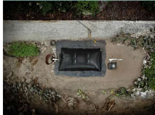
Sistema 12 Area Required: 3.4 X 7.7 m Biogas: 3.3 m 3 /day*
