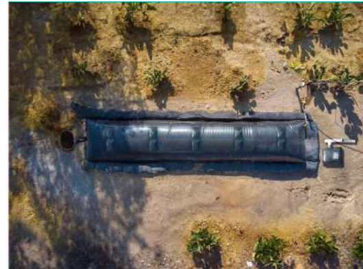
Sistema 30 Area Required: 3.4 X 15.7 m Biogas: 6.7 m 3 /day*
