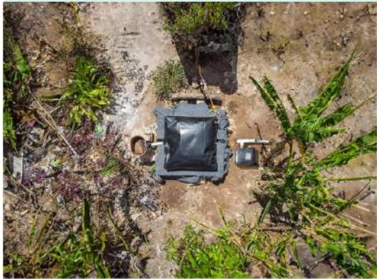
Sistema 6 Area Required: 3.4 X 5.4 m Biogas: 1.7 m 3 /day*
