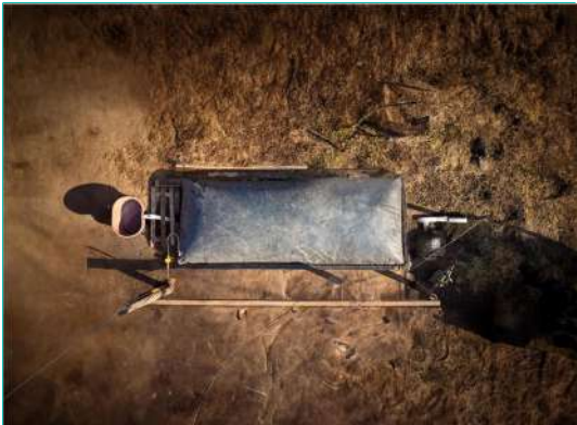
Sistema 16 Area Required: 3.4 X 9.7 m Biogas: 4.8 m 3 /day*
