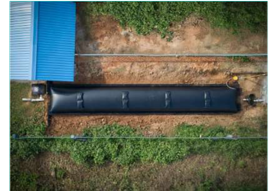
Sistema 40 Area Required: 3.4 x 20.7 m Biogas: 13 m 3 /day*
