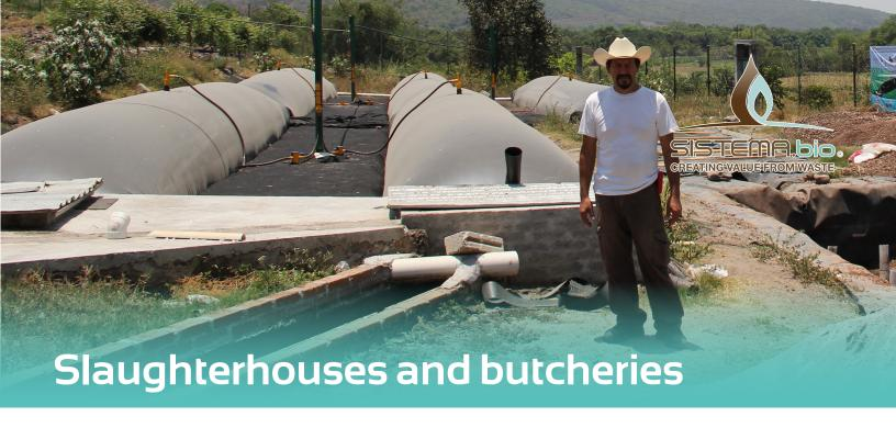
**Sistema.bio**® is a waste treatment system for small and medium scale slaughterhouses, especially for blood, manure, and fat treatment. The byproduct of this process is renewable energy -biogas- and biofertilizer. The biogas can be used for water heating, meat cooking, or for running small engines.
